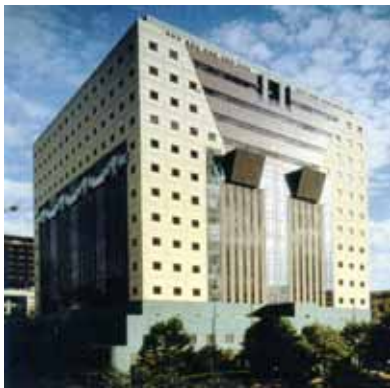
Michael Graves and Partners. Portland, Oregon USA. Offices 1979-82. Post Modern Façade wallpaper over early modern interior.
